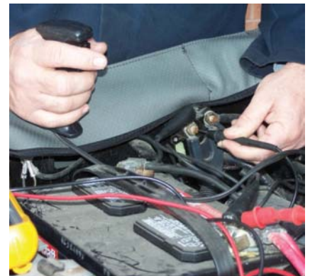
P4-6 If the reading is out of specifications, test at the next connection toward the battery. In this instance, the next test point is the starter side of the relay.
