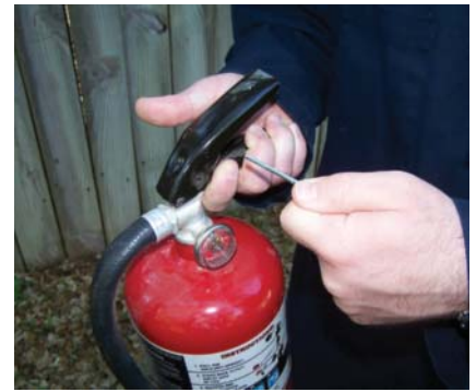
P1-3 Pull the safety pin from the handle.
