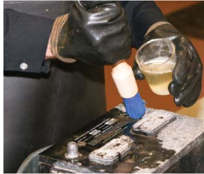
P9-11 Brush the solution over the battery case. Be careful not to allow the solution to enter the cells of the battery.
