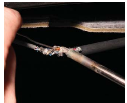
PS7-12 Splice the drain wire with a clip and solder.
